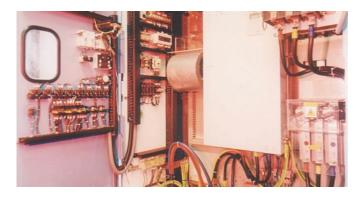
Logicon selected the Mitsubishi Electric Meltrac MT A140E inverter, because of its small physical size and the option to have either the "auto energy saving facility", or the "sensorless vector control" which gives 150% torque at low speed which is ideal for their purposes.
